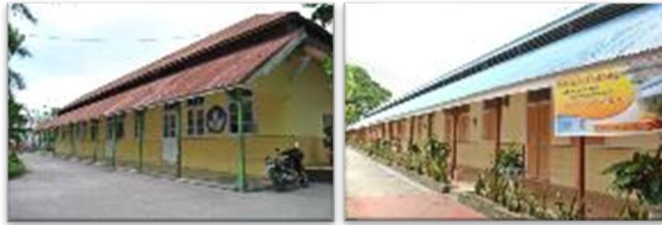
Figure 13. The Building of SMAN 1 (former HCS) and that of SDN 061 (former HIS) (Source: The Writers, 2020)
